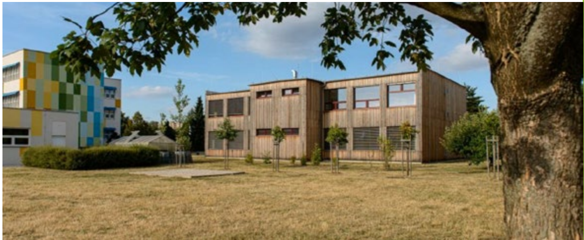
Figure 5: Modular primary school in Petrovice, Czech Republic
