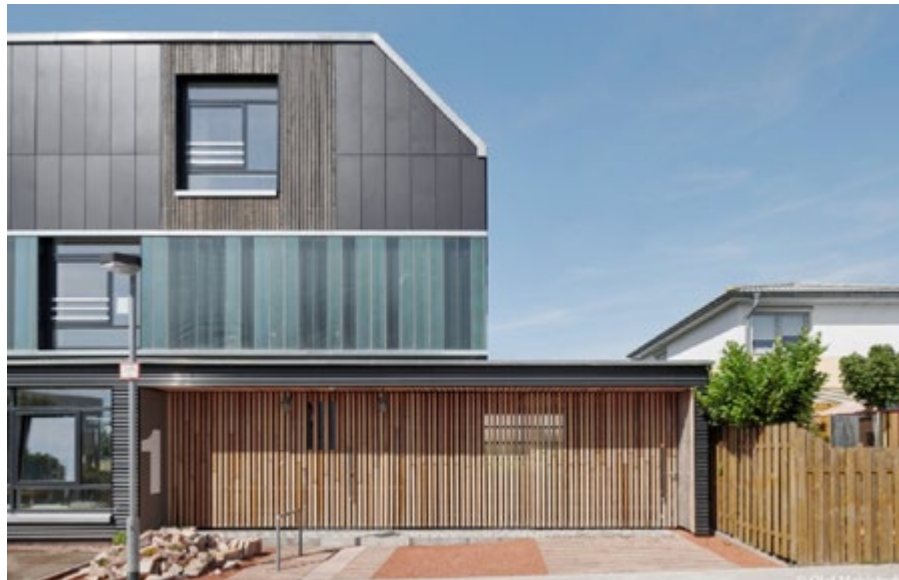
Figure 12: Recyclinghaus in Kronsberg, Germany
