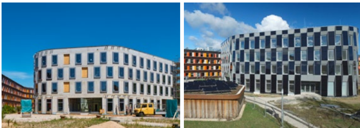
Figure 9: Building of UBA – new construction with recycled concrete
