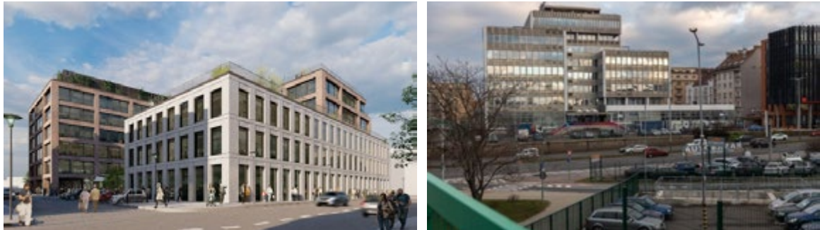
Figure 7: Office building Mercury: new and existing building
