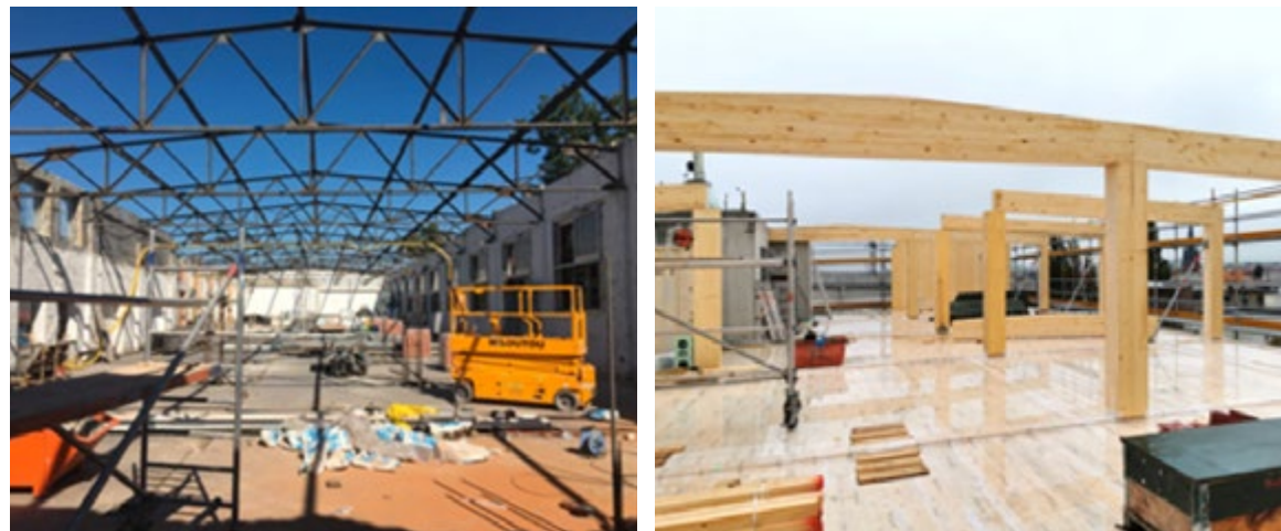
Figure 8: Renovation of the existing building and extension in timber construction
