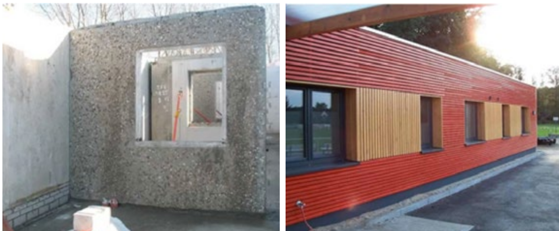
Figure 10: Sports House Kolkwitz – reuse of reinforced concrete slabs
