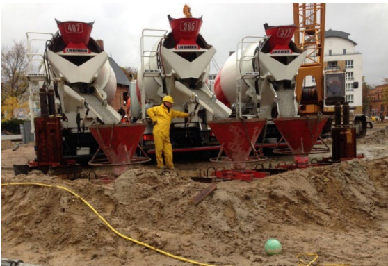
Placing of the R-concrete
