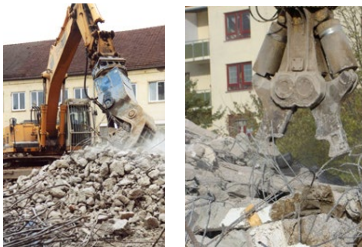
Fig. 10. Demolition grab (left), scrap shear (right)
