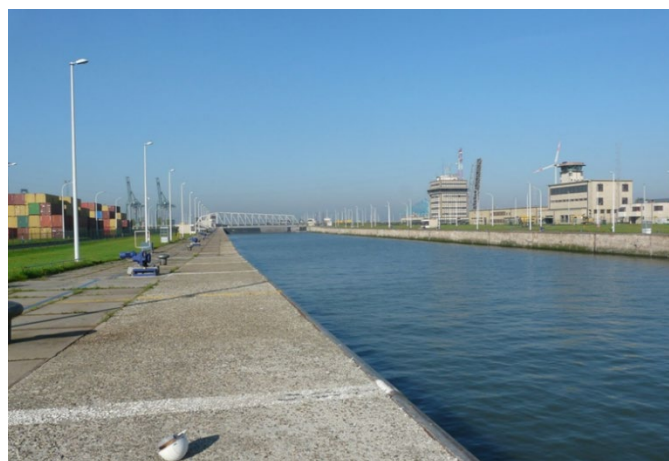
Fig. 37. View of the Berend-recht lock in the port of Antwerp built with recycled coarse aggregates (Image source: Jeroen Vrijders, Belgian Building Research Institute)
