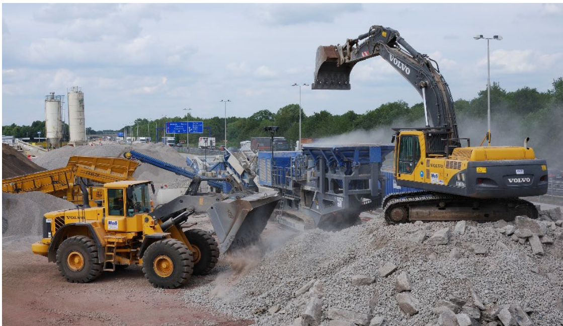
Fig. 13. Mobile processing plant during crushing of concrete recovered from a highway
