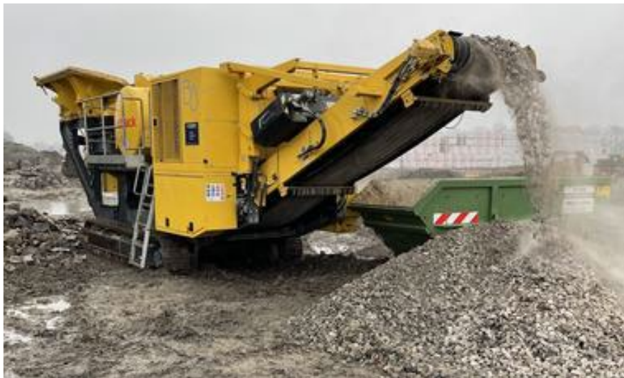
Fig. 20. Jaw crusher during crushing of building rubble [14]
