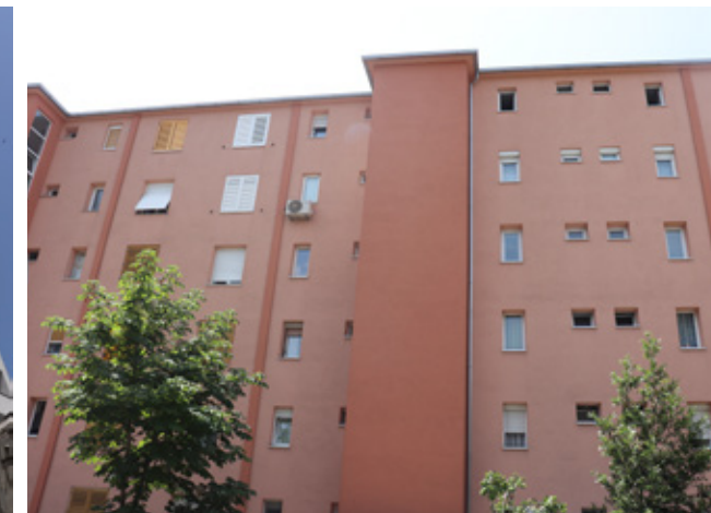
Drage Gervaisa 24, Rijeka – renovated buildings in the Street Drage Gervaisa, Rijeka (resource: The Environmental Protection and Energy Efficiency Fund)
