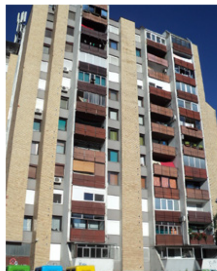
Sjenjak 101, Osijek – building before renovation (resource: Krešimir Ižaković, condominium representative)
